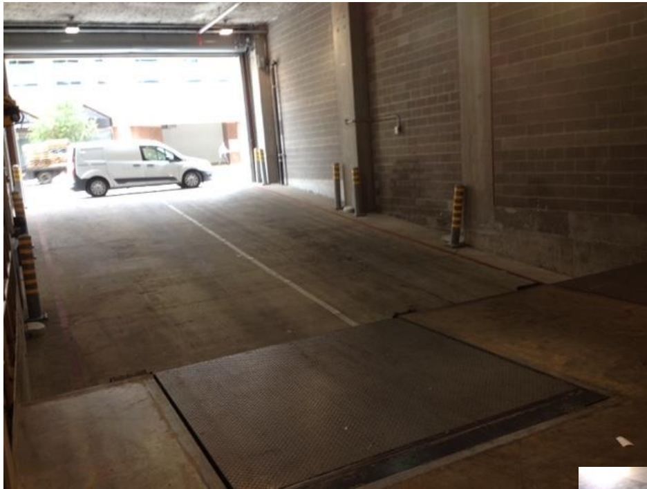
View of 2 dock bays
