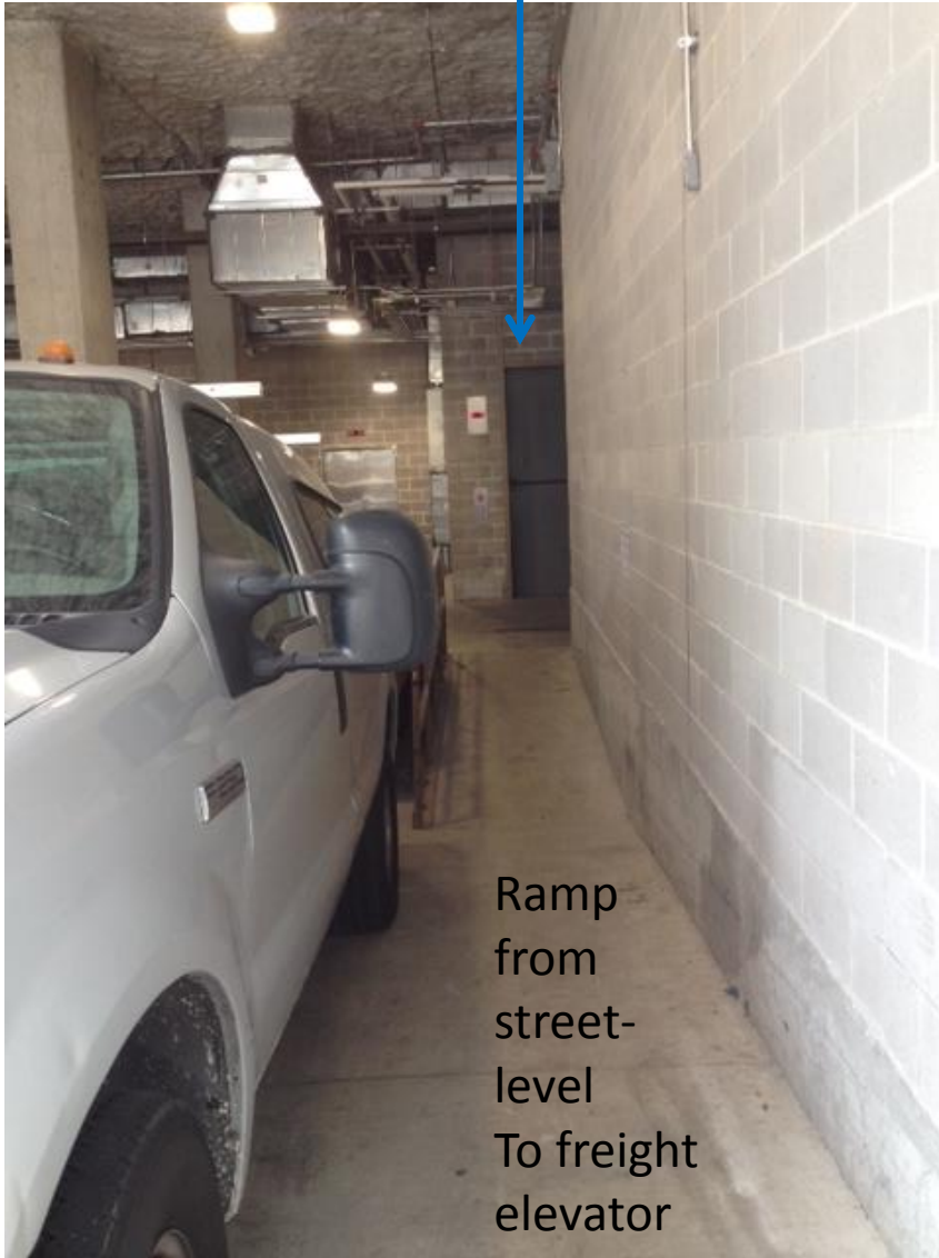
1 of 2 freight elevators
